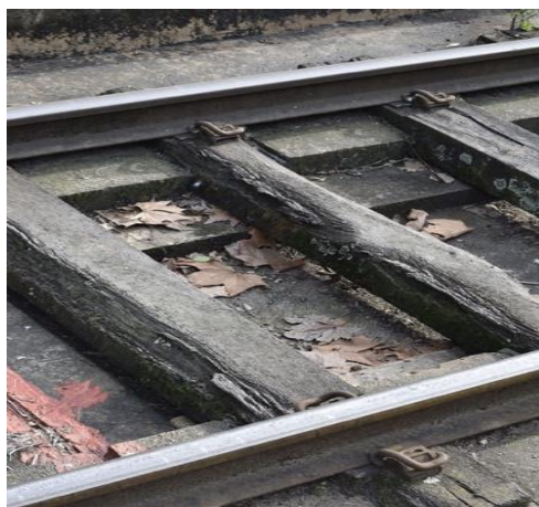
Image 5. Sleepers of Railway tracks
